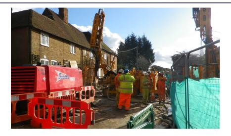
The A2163 road through Leeds, near Maidstone, Kent collapsed during the winter of 2013/14 revealing a large void below the highway and also voids extending beneath adjacent properties.
